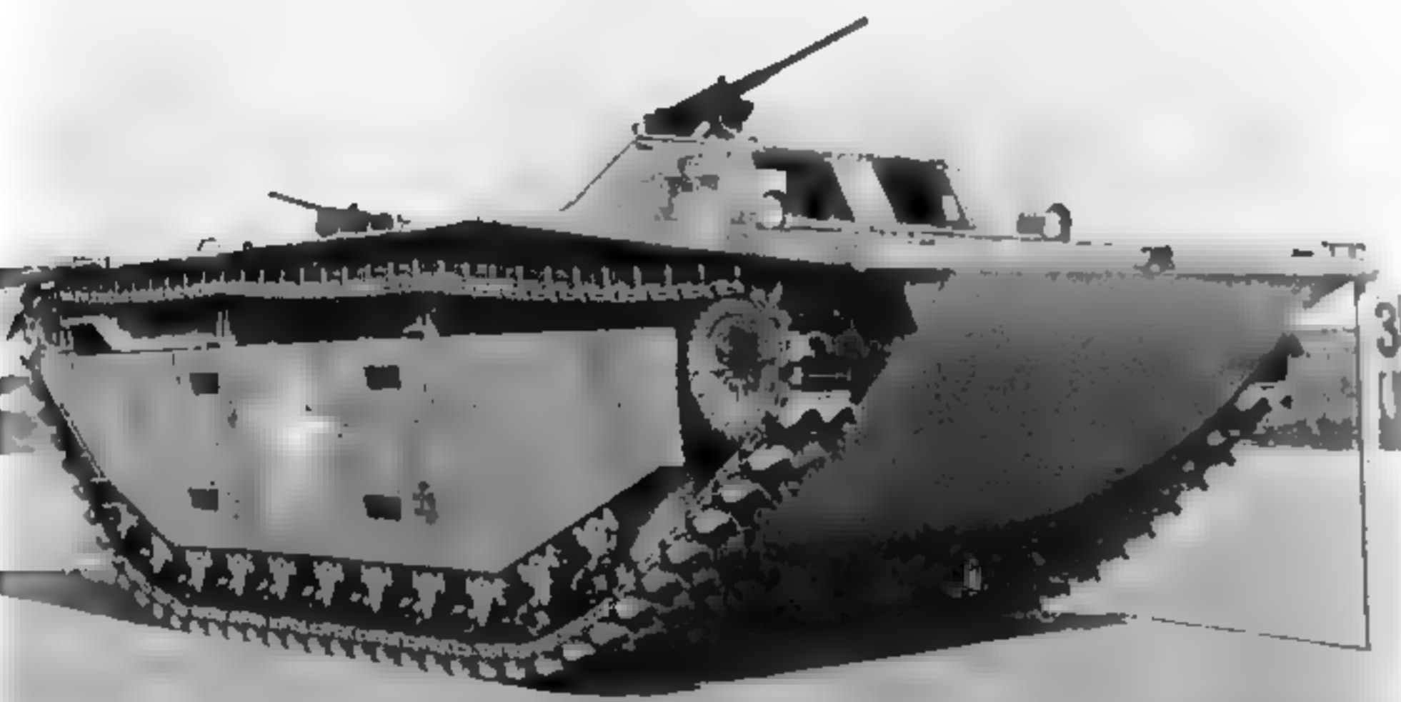
The LVT (2) shown here is an early production model, based on the four step pockets in the side. Later vehicles had only two per side. The uneven height of the machine gun is a result of the discontinuous ring, the short forward section was mounted higher than the side and rear section. (National Archives and Records Administration photo)
